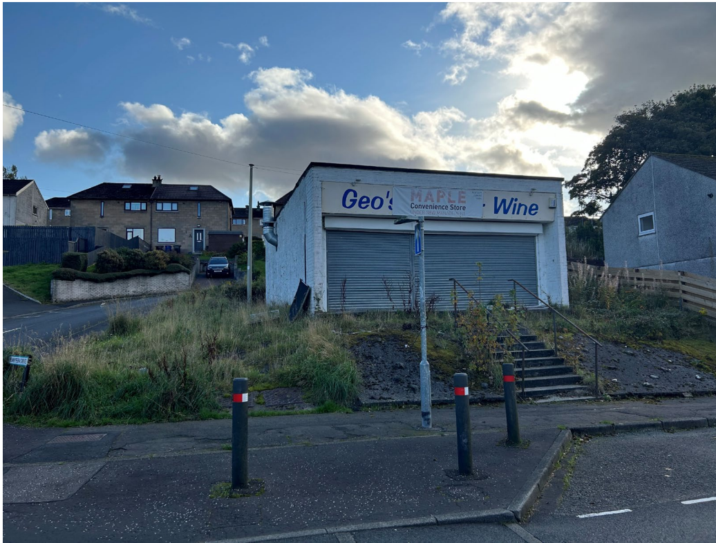
View of the front elevation of 58 Maple Road, Greenock
